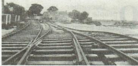
Flooding was a common occurrence until the river was diverted. Below - The undermined railway lines.
